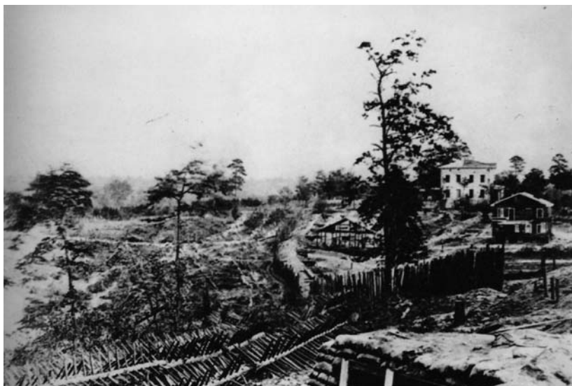
Palisades and chevaux-de-frise in front of the Potter House, Atlanta, Georgia (NA 111-13-726).
